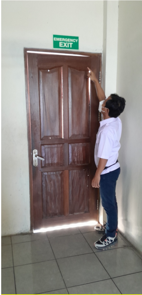
Inspeksi Emergency Exit
